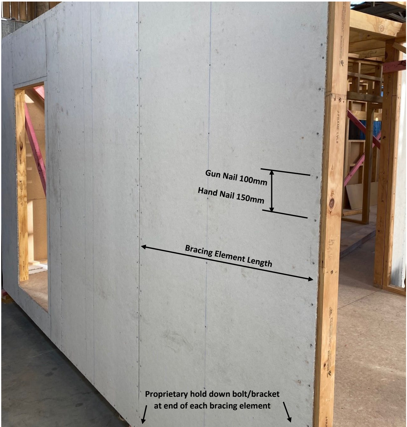
DIAGRAM 5 – Bracing Board fixings
